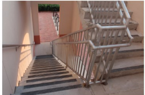
Durlach Industries' SunSeeker contract calls for stairs bearing Wooster Type 231 BF, Supergrit safety treads. A heat-treated, corrosion-resistant, extruded aluminum base finished in satin lacquer frames a tread insert cast with diamond hard aluminum oxide for long life under heavy pedestrian traffic. The 3-in. wide, 1/4-in.-thick non-slip treads ship cut to length, ready to replace temporary wood slats used for construction traffic.
